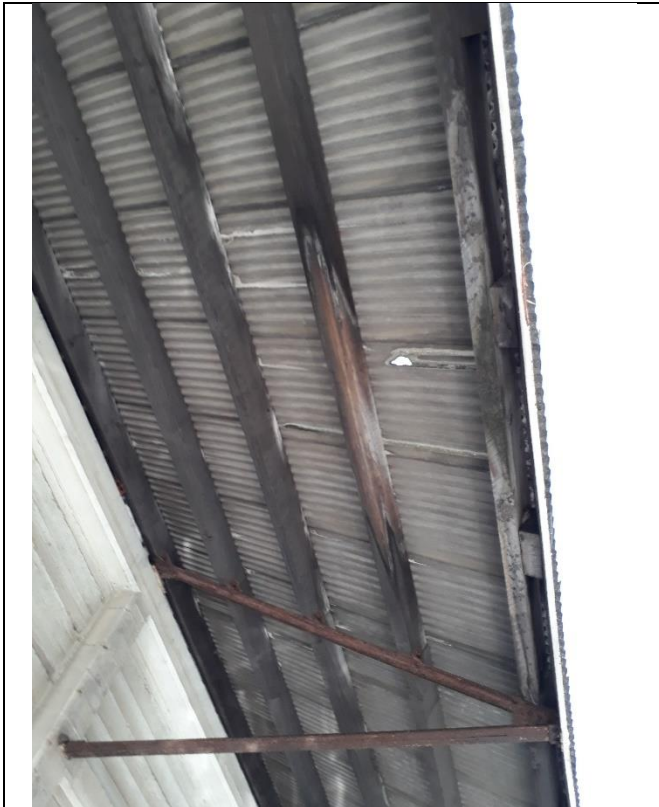
Super six roof overhang seen from below Water marks, holes and damaged edges are easily visible
