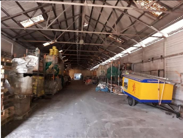
Interior of Qa Shed
