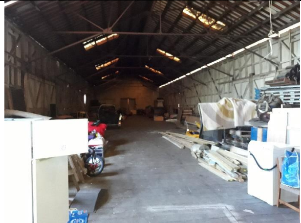
Interior of R Shed
