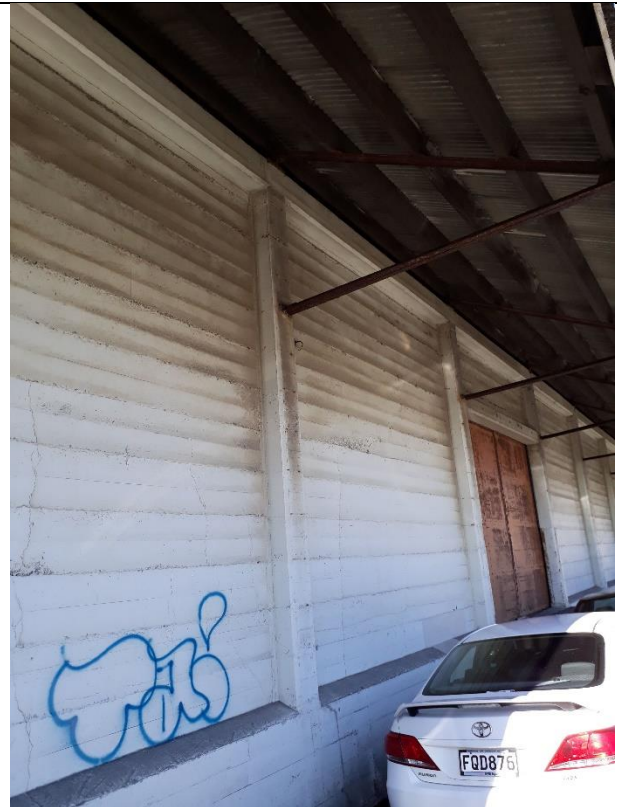
Dust gathered on an exterior wall
