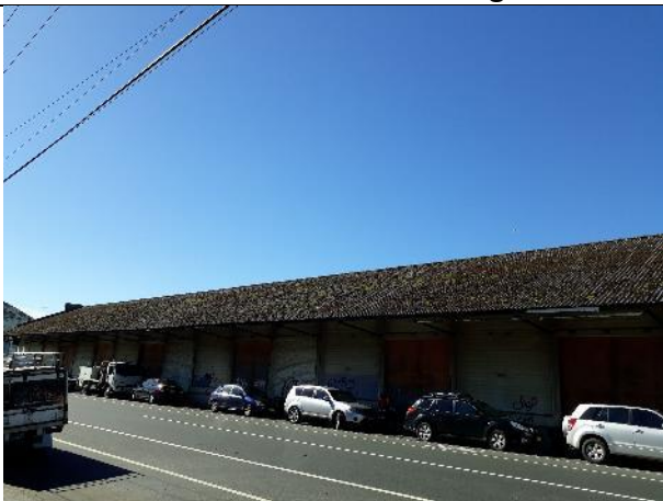
Exterior of R Shed Cars parked under the roof overhang
