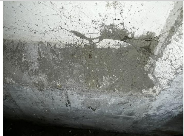
Dust on internal wall ledges
