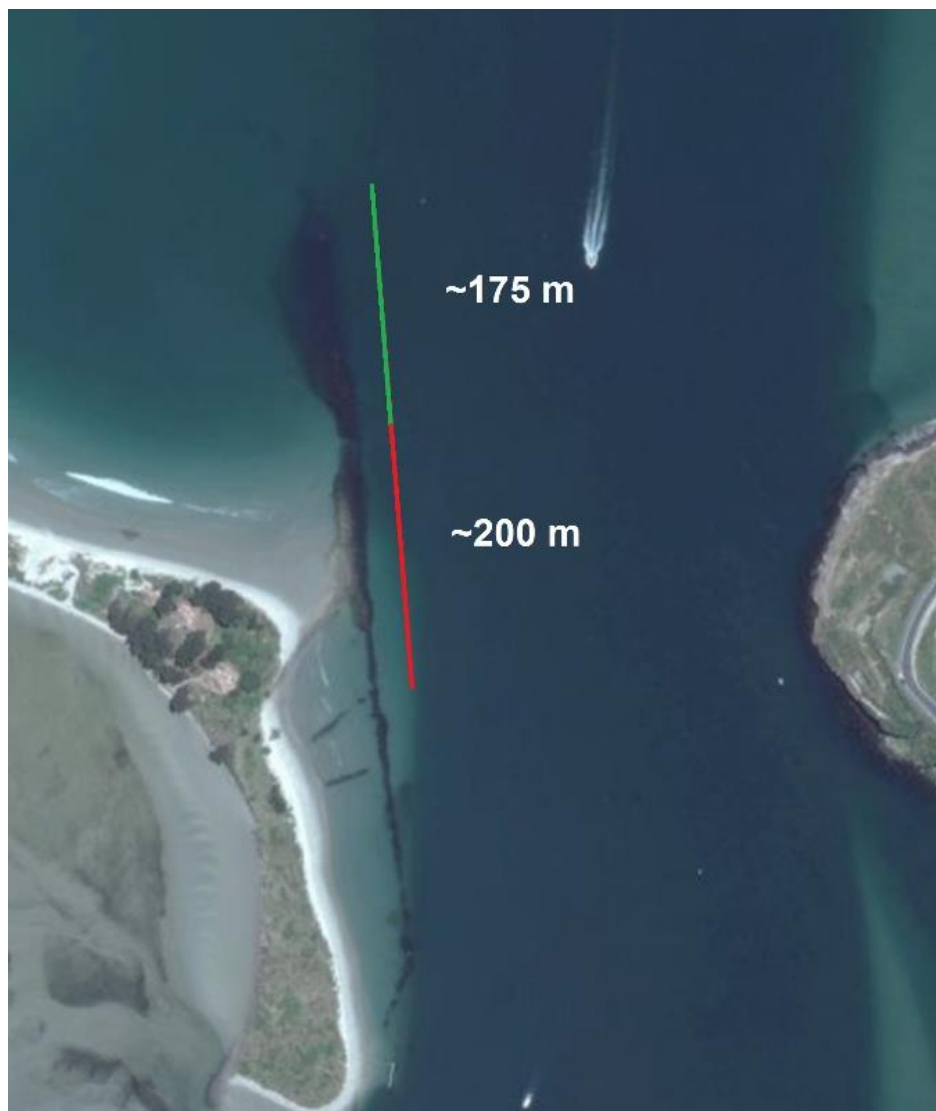
Figure 4.1 Aerial view of the Long Mac structure with definition of segments raised to +1.1 m MSL (highest astronomical tide).
