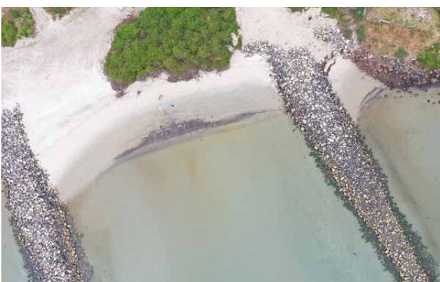
This aerial view provides an insight into the degree of engineering involved in the breakwaters' design and build. Each of the three groynes is anchored well back into the beach to protect sand from being washed away by the wind and tides.
