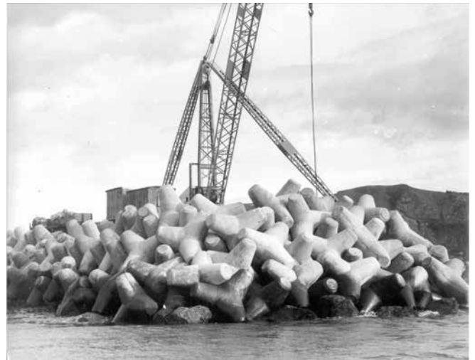
These 5-tonne concrete tetrapods were placed on the end of the mole about 60 years ago, but were no match for the ocean and tides.
