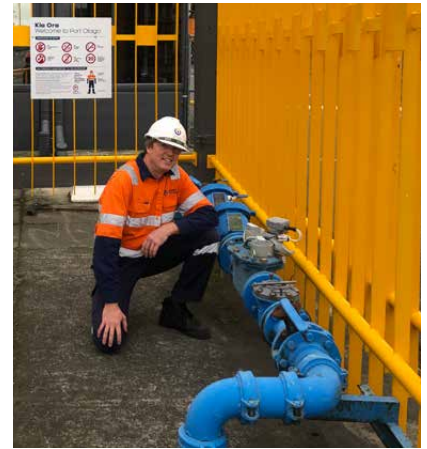
Water monitoring on the Port Chalmers terminal stepped into the modern age last year, with the installation of electronic water meters by the city council. Port Otago Infrastructure Asset Engineer Jon Visser says the meters enable the port to detect and stop leaks much sooner.
