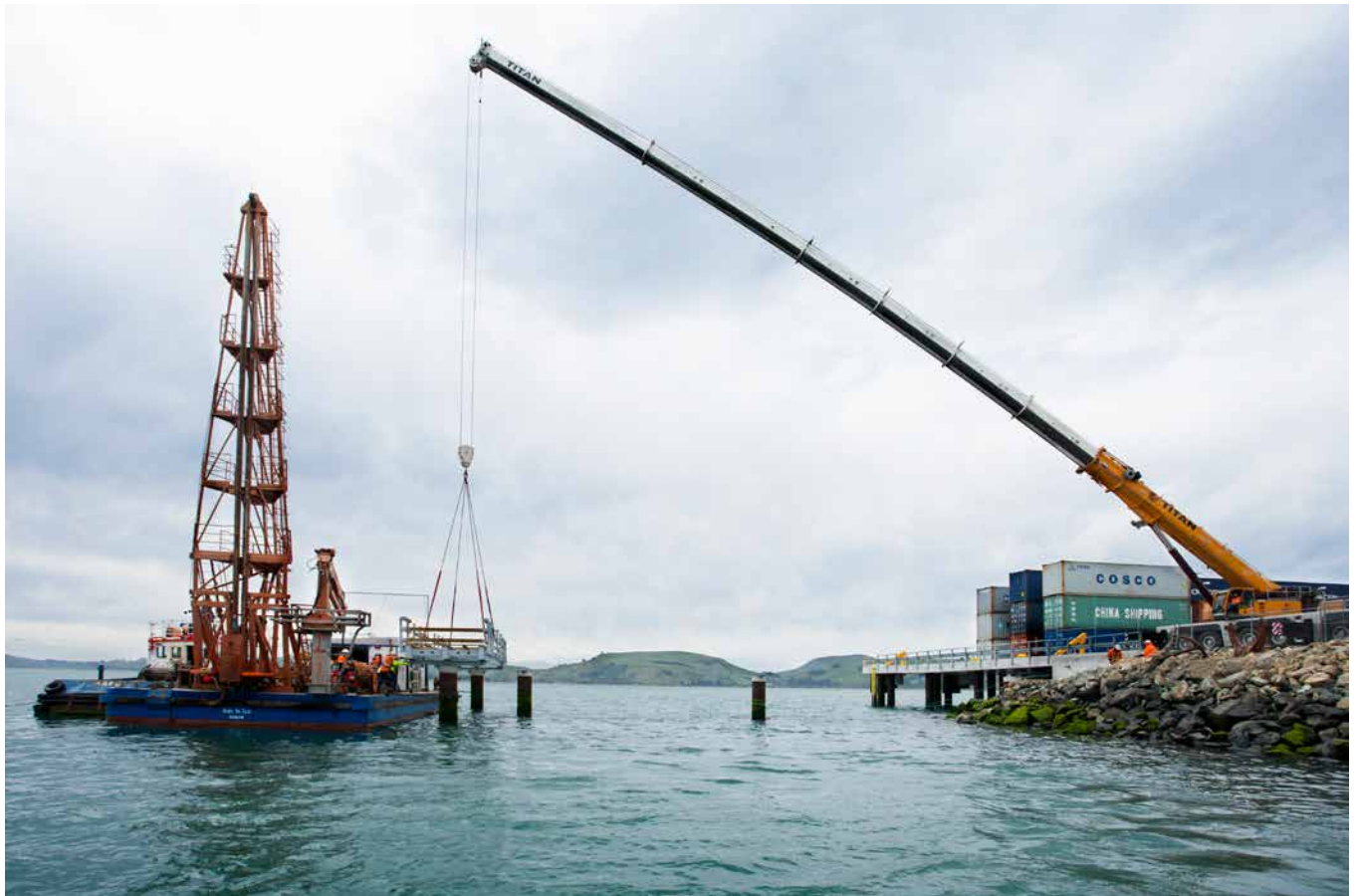
A massive 250-tonne crane was brought down from Christchurch (there was not a big enough crane in Otago) to lift the jetty's four sections into place. This photo shows the largest section – the "T" (17m long, 3.5m wide, 8 tonnes) – being positioned into place. Photo courtesy Brian Corson
