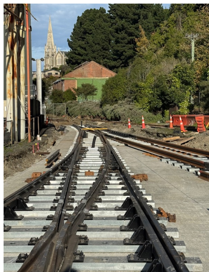
The rail pad's three new sets of southern turnouts, with the Sims building in the background.
