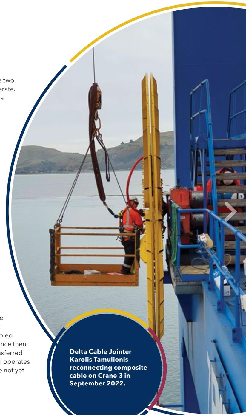
**Delta Cable Jointer Karolis Tamulionis reconnecting composite cable on Crane 3 in September 2022.**
